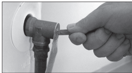
Figure 50: T&P Relief Valve.
