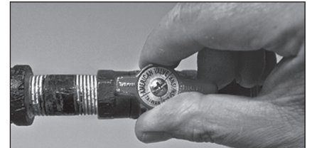
Figure 56: Gas valve in "on" position.
