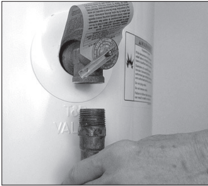
Figure 13: Removing the T&P Relief Valve discharge pipe.
