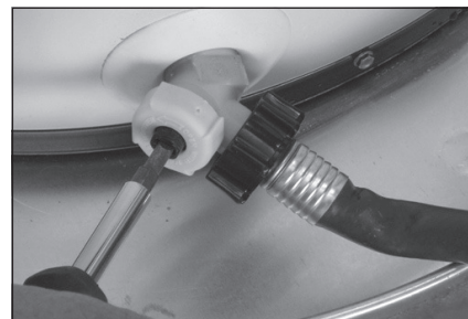
Figure 12: Draining the old water heater.
